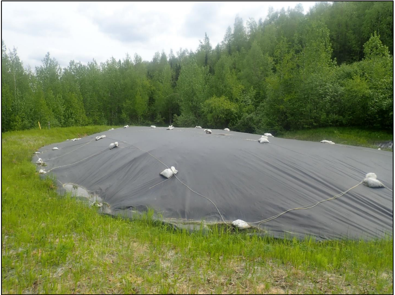
Photograph 2-7. Overview of lower soil stockpile with cover and sandbags intact, 6/6/2024.
