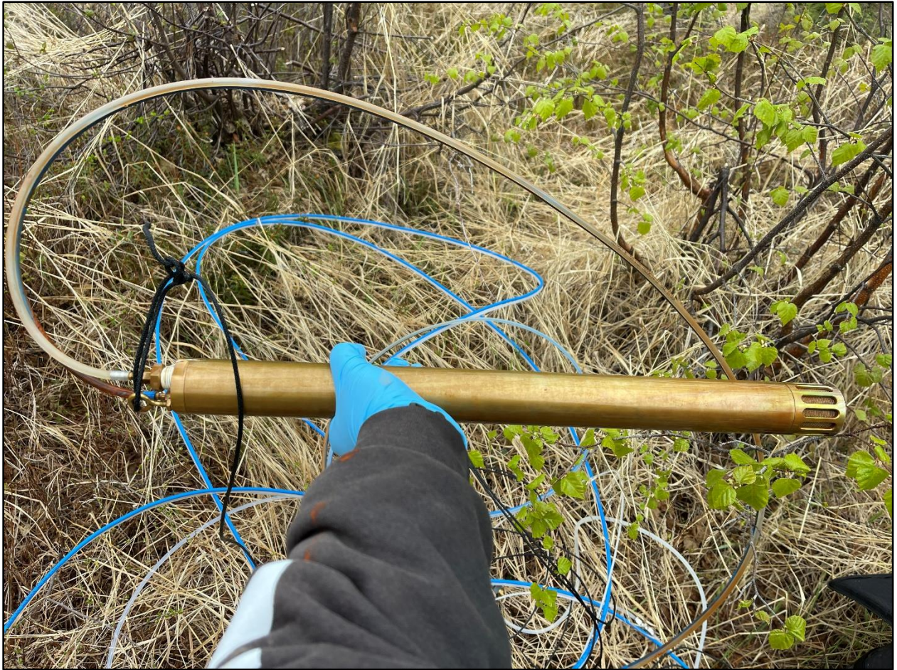
Photograph 2-9. Discoloration and rusting of bladder pump on MW50, 6/2/2024.
