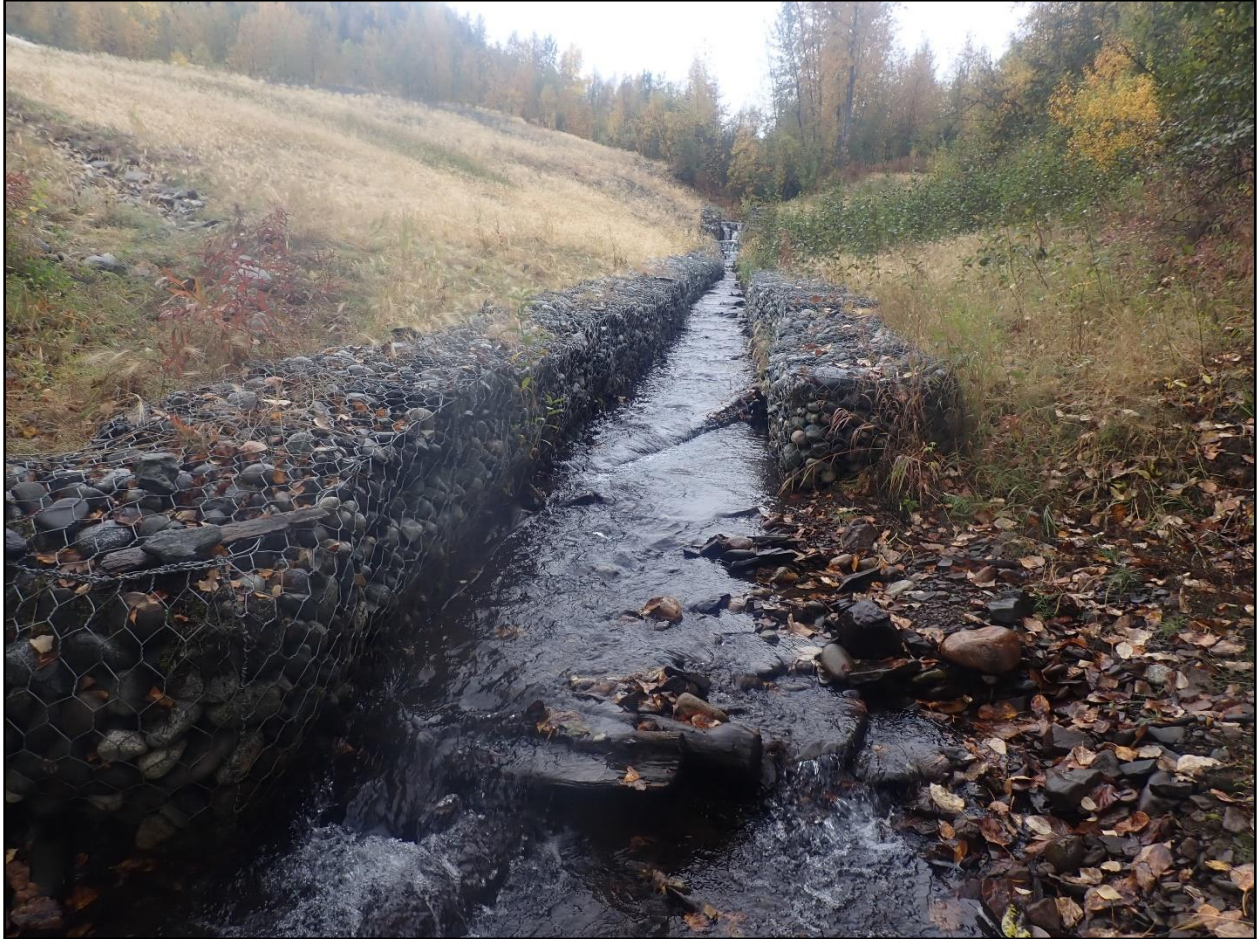
Photograph 2-2. Upstream view of Red Devil Creek along the engineered and stabilized section, 9/12/2024.
