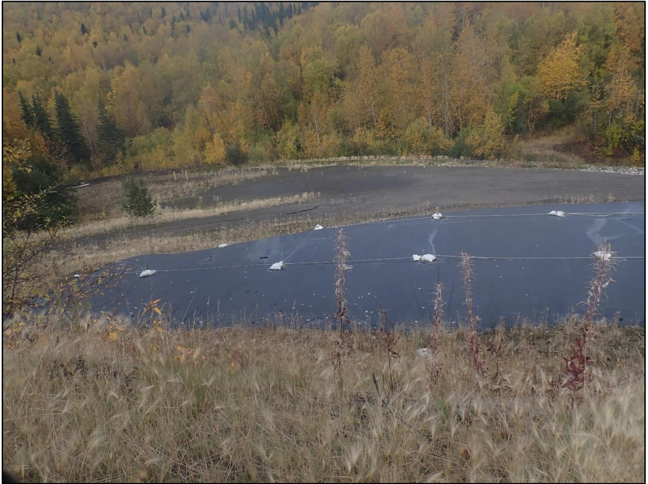
Photograph 2-4. Engineered slope and covered stockpile, 9/12/2024.
