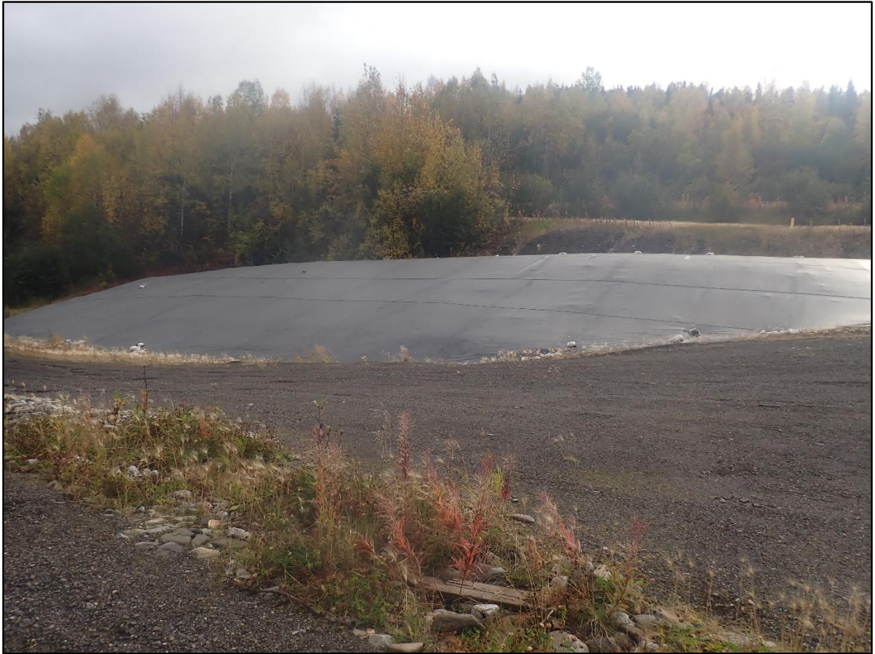
Photograph 2-7. Engineered slope and covered stockpile, 9/12/2024.
