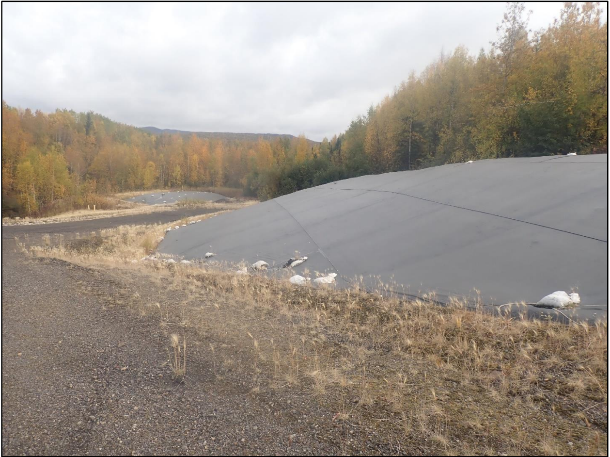
Photograph 2-5. Engineered slope and covered stockpile, 9/12/2024.
