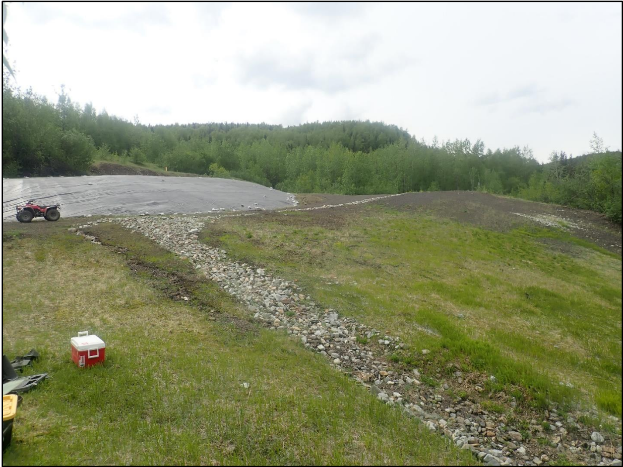
Photograph 2-6. Overview of engineered slope and covered stockpile, 6/6/2024.
