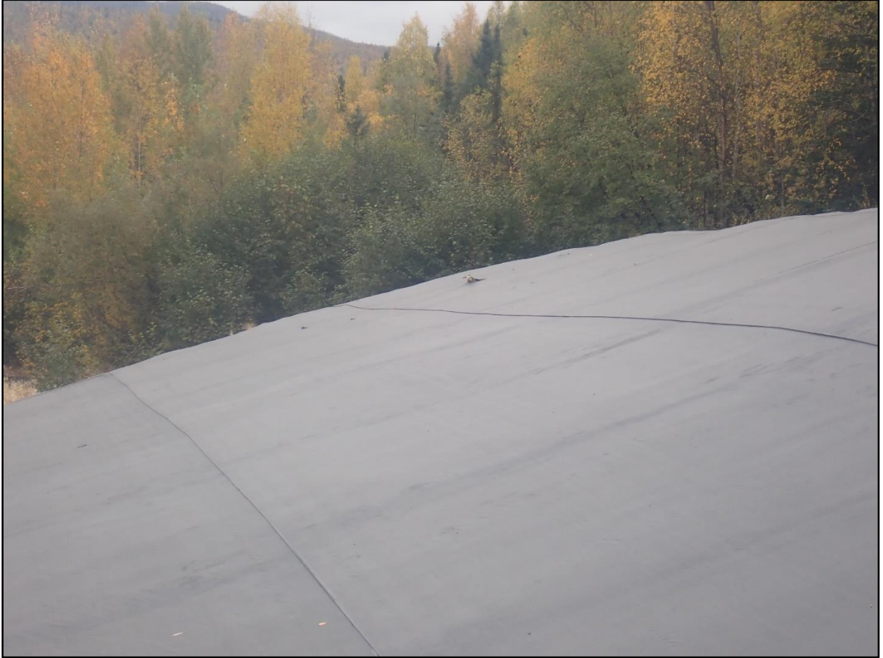
Photograph 2-6. Engineered slope and covered stockpile, 9/12/2024.
