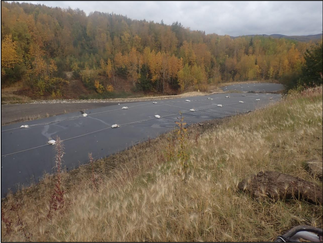
Photograph 2-1. Engineered slope and covered stockpile, 9/12/2024.
