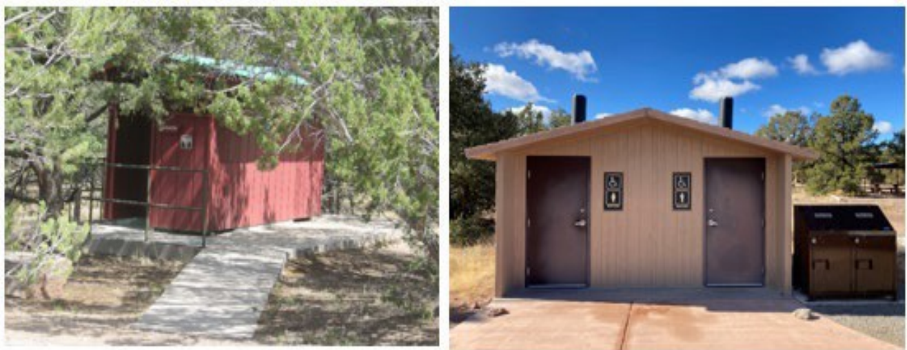
Figure 12: 2022 Vault Toilet Replacement
