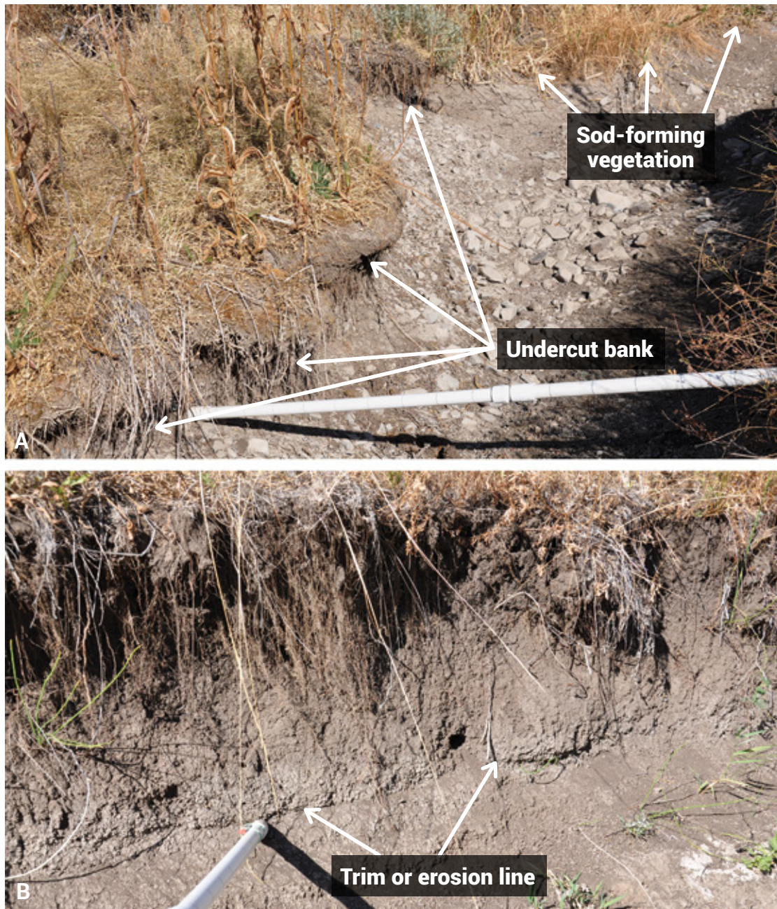
Figure H.1. A. The scour line is delineated by the lower limit of sod-forming vegetation and the ceiling of undercut banks. B. The scour line coincides with the trim or erosion line on bare banks. This erosion line marks the water stage during baseflow conditions and coincides with the ceiling of undercut banks elsewhere in the DMA.
