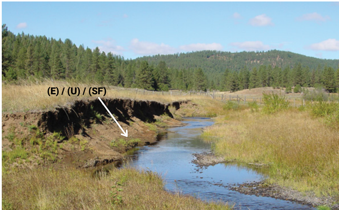
Figure H.9. The left bank in this photo is erosional (E) and uncovered (U) with no vegetation, rock, or wood. The lower two-thirds of the bank has accumulated loose aggregates of soil, or slough (SF), which likely will be removed from the bank during high streamflow.
