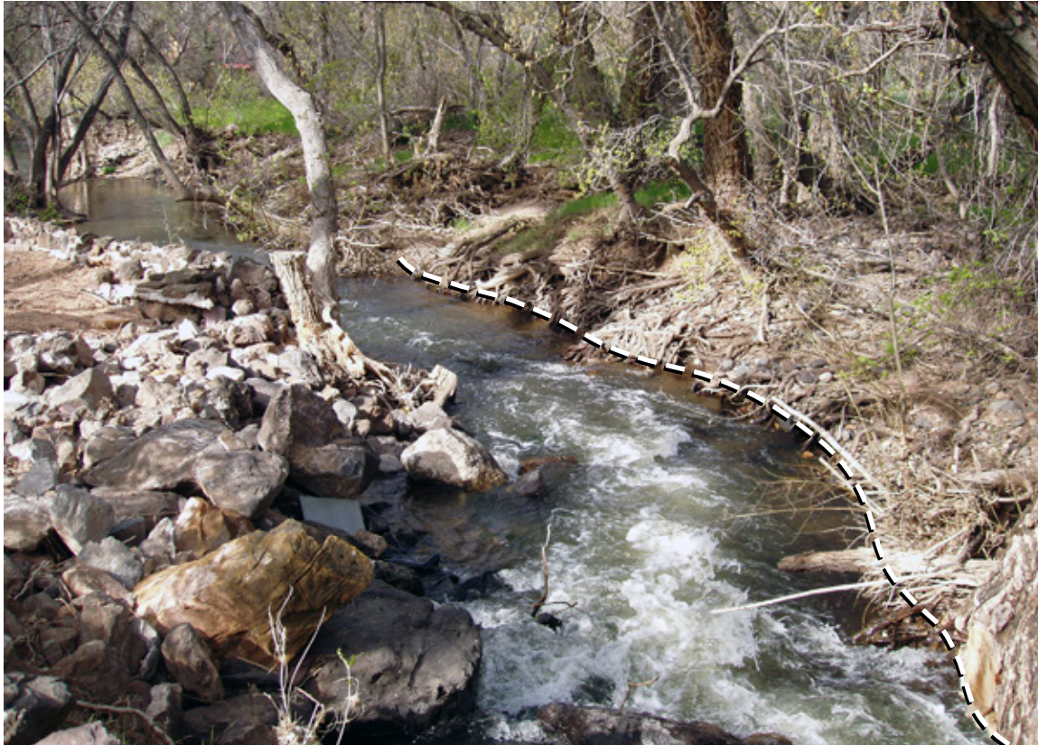
Figure D.18. Exposed live shrub or tree roots at or above the scour line are part of the greenline.
