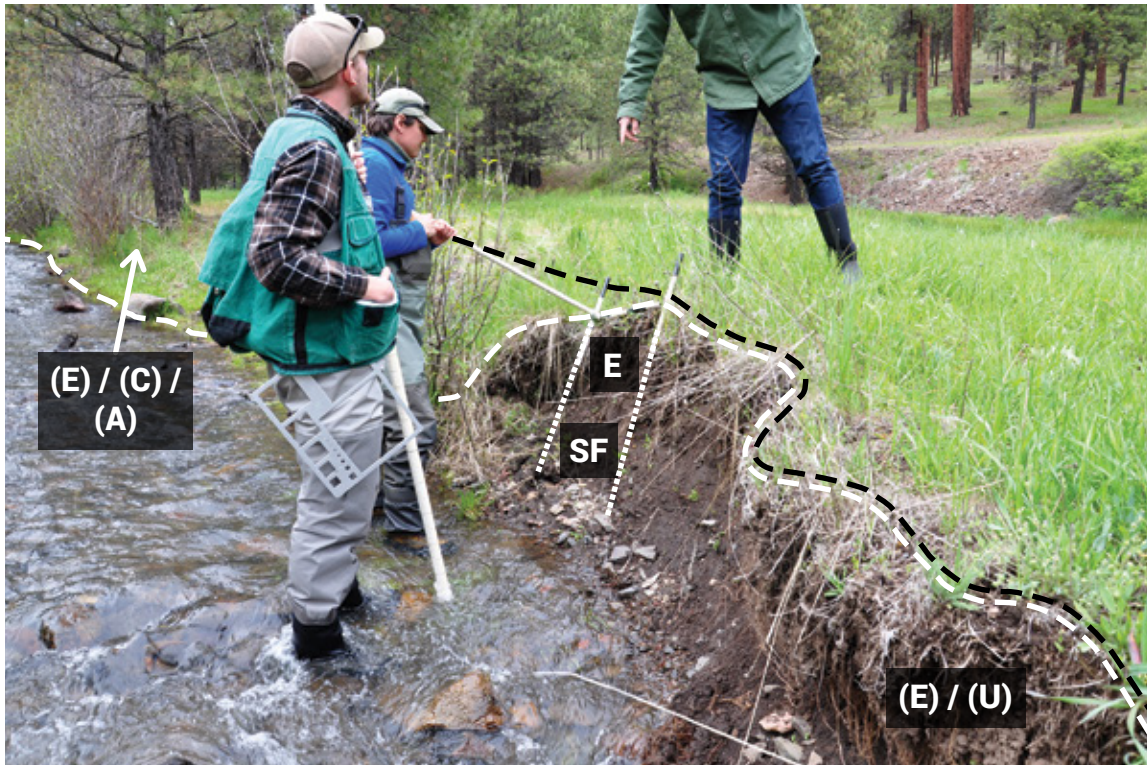
Figure H.11. The water surface is at the scour line in this photo. The bank in the background is erosional (E), covered (C), and absent (A). The bank in the foreground is erosional (E) and uncovered (U). The upper part of the bank is nearly vertical and eroding (E), while the lower part of the bank has an accumulation of slough (SF). It is not uncommon to have more than one instability feature in the streambank stability quadrat. In this case, the instability feature could be listed as either eroding (E) or slough (SF).
