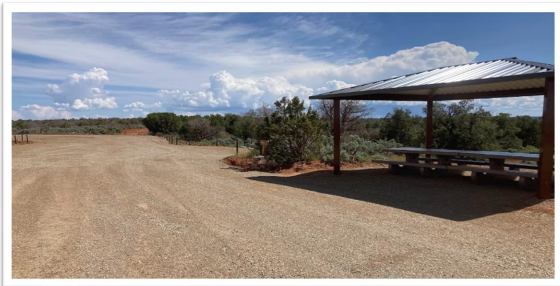
A new road, parking lot, picnic shelter, restroom, and interpretive trail were constructed at the Painted Hand Pueblo public site in 2023.
