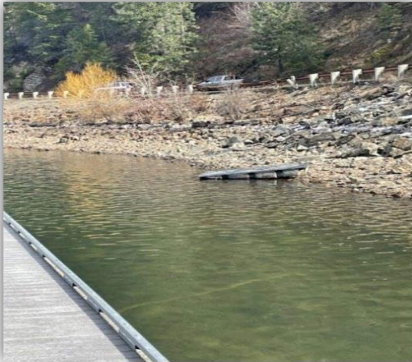
Figure 9: Dislodge dock float tub at Mineral Ridge Boat Launch
