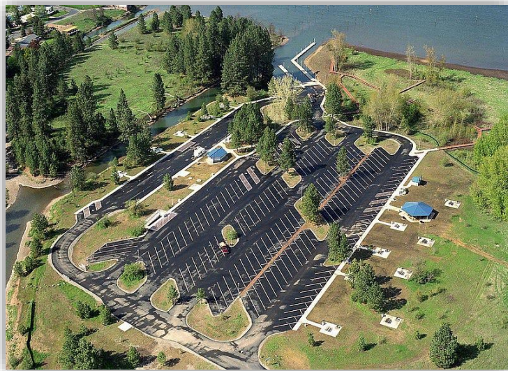
Figure 1: Aerial View of Blackwell Island
