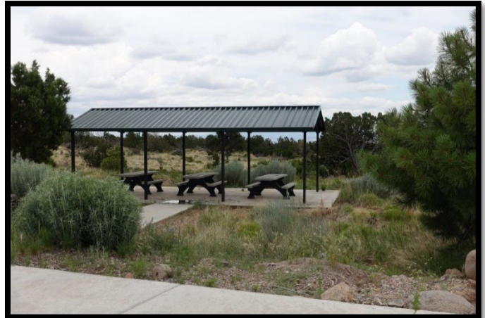
Group picnic area and ABA-accessible path at Veterans' Memorial Overlook.
