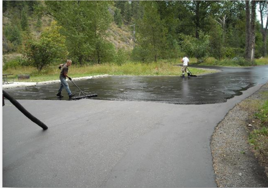
Figure 4: 2009 sealcoat, striping, and pavement repairs.
