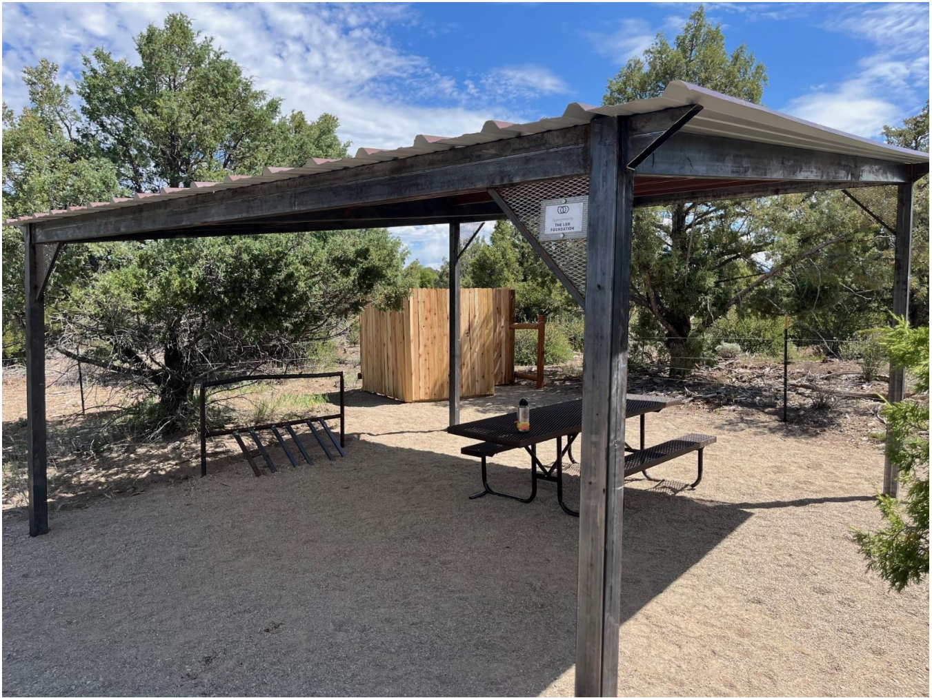
The Aqueduct parking area benefitted from improvements driven by local partners.
