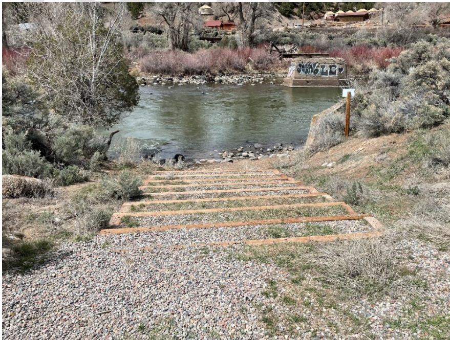
State Bridge Ramp #2
