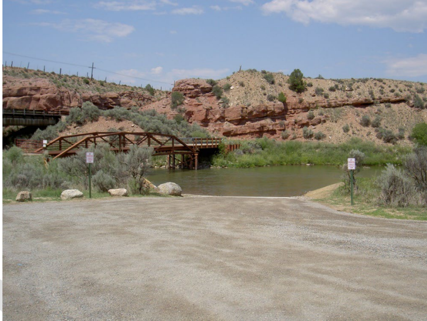
Two Bridges Site – Improved Boat Ramp
