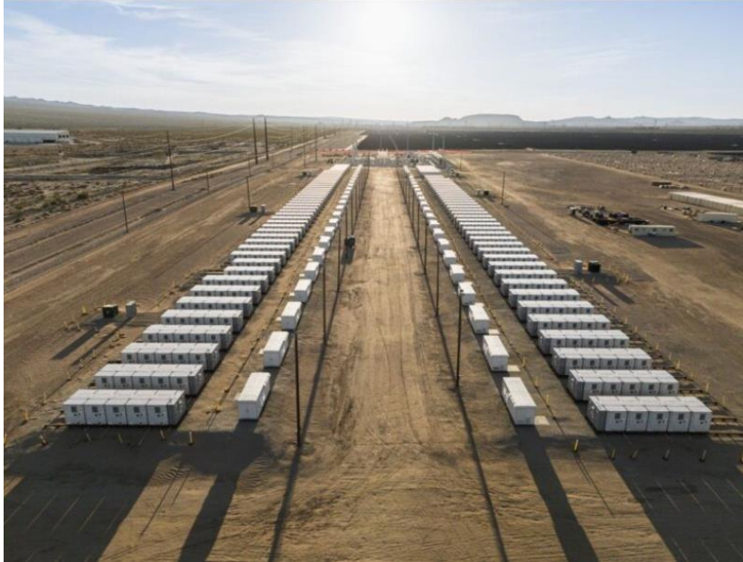
Figure 6 Typical BESS
