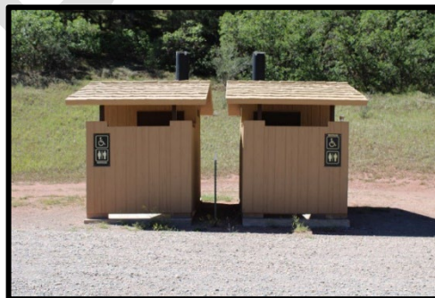
Figure 7 Specie Creek Day-Use Area's vault toilets managed under LLCOS05000
