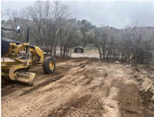
Saul's Meadow Campground Construction
