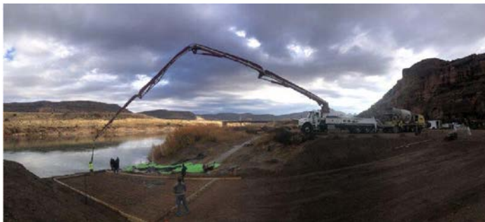
BLM Maintenance Assists with Ramp Improvements
