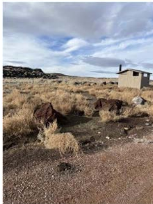
Facilities maintenance needs addressed
