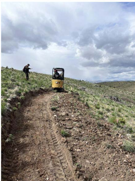
BLM helps guide machine operator building trail
