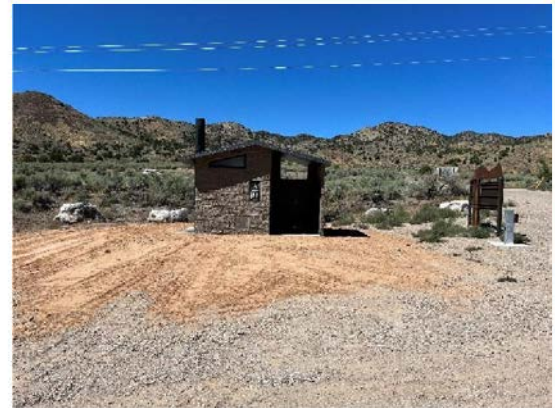
New Restroom Installed at Hanging Rock Campground
