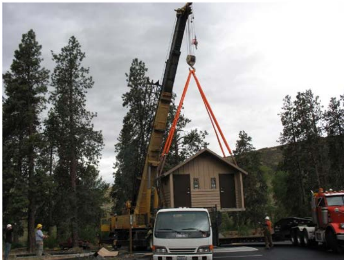
Contract to install new double outhouse in 2024
