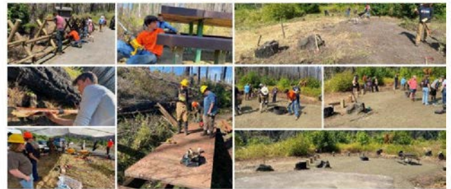
Day Use Site and Trailhead Repair
