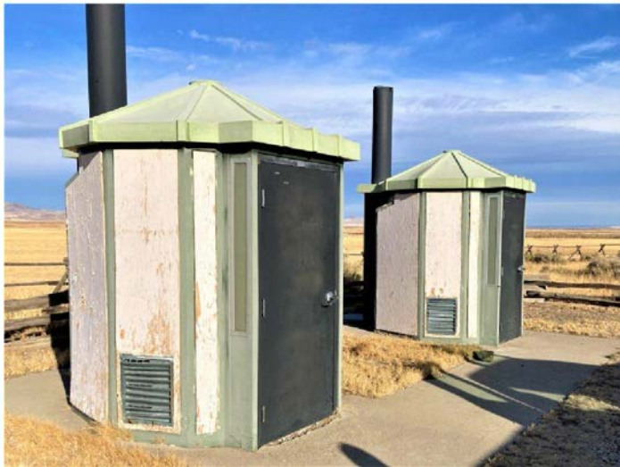
Hart Bar vault toilets to be replaced.
