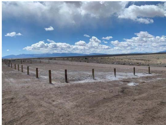
Completed parking area for UFO skip site.
