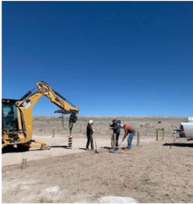
BLM Staff Working on Parking Lot
