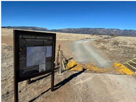
Finished informational Kiosk
