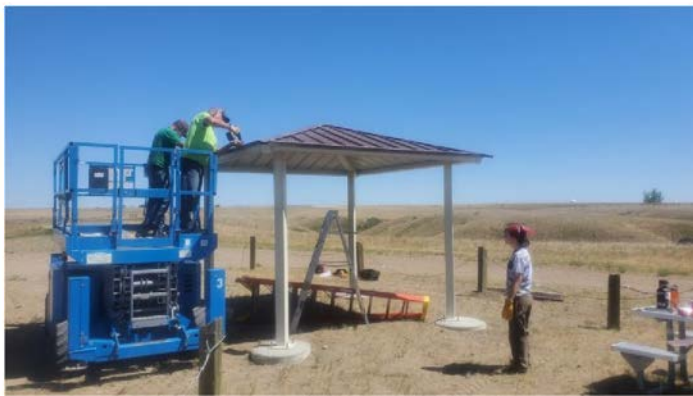
Assembling Picnic Structures
