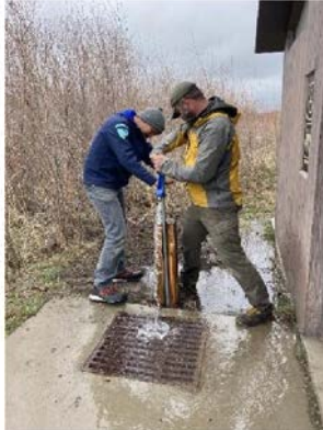
BLM Recreation Staff Repair a Potable Water Well
