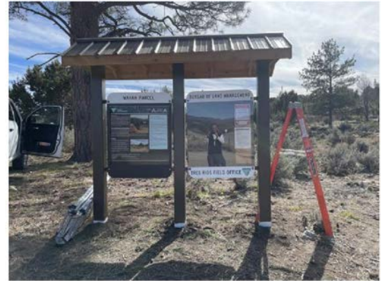
Mahan Kiosk Installation
