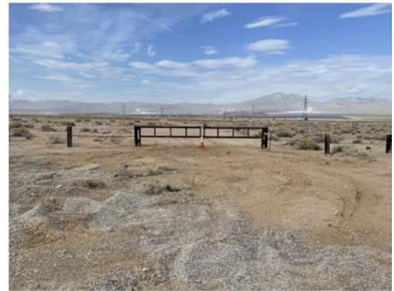
New Access Gate
