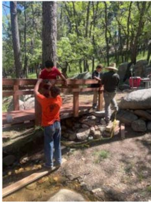
Scouts Work to Install Handrails
