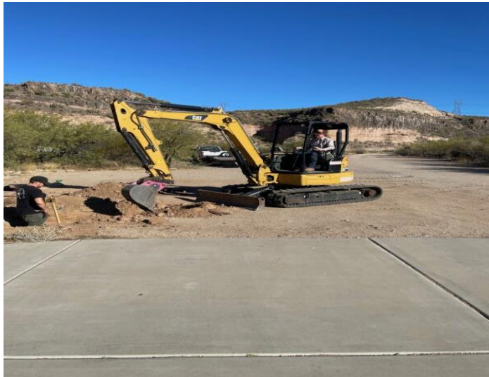
Excavator Exposes Waterline
