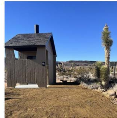
ADA Compliant Ramp at Pakoon Springs
