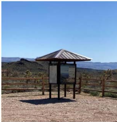
Pakoon Springs Trailhead Kiosk Roof
