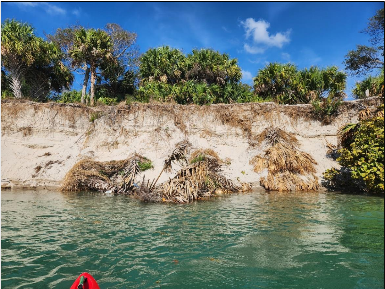
Erosion along the ONA's Indian River Lagoon Shoreline showing loss of vegetation (collapsed cabbage palms and Seagrape)
