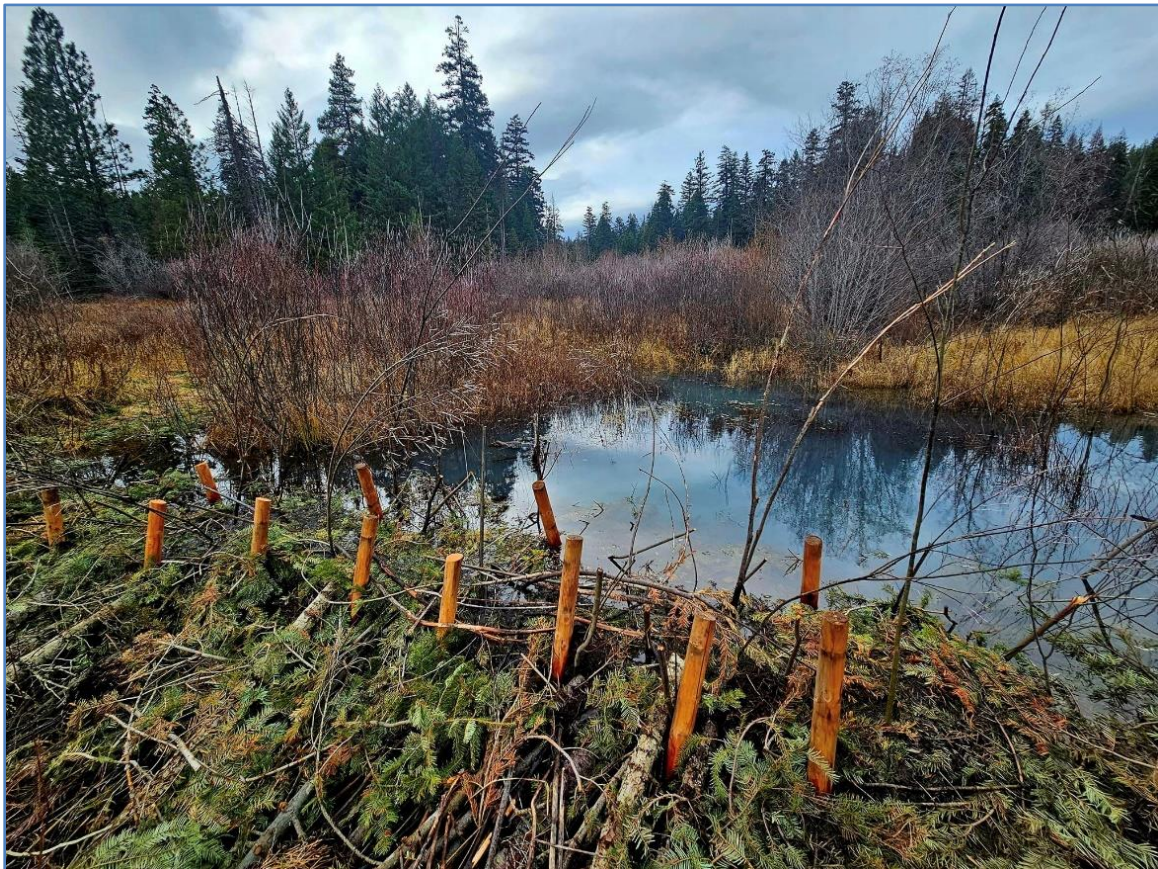
Beaver Dam Analog (BDA) structure in CSNM
