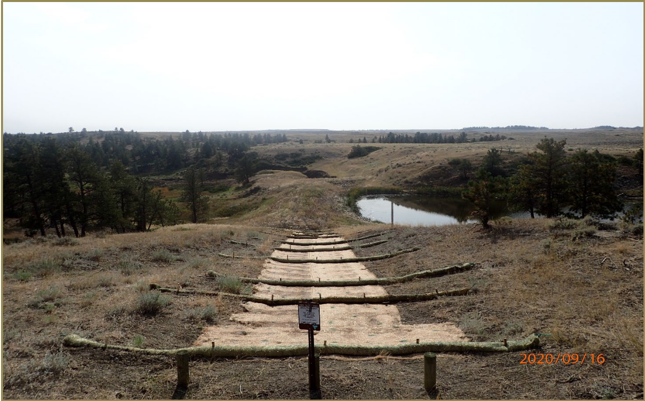
Butch Reservoir Road Reclamation
