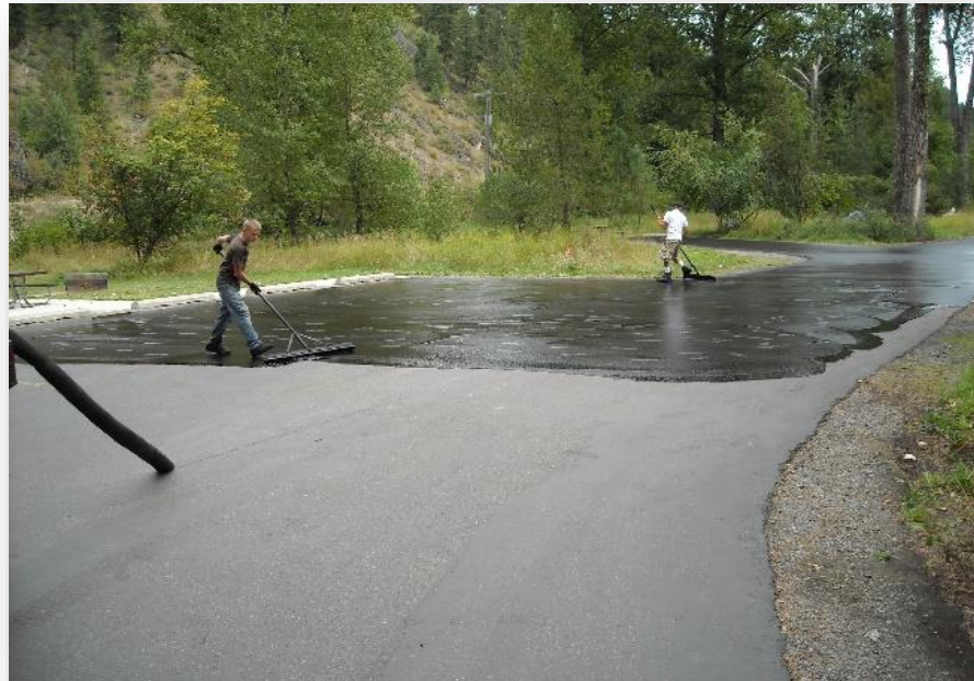
Figure 4: 2009 sealcoat, striping, and pavement repairs.
