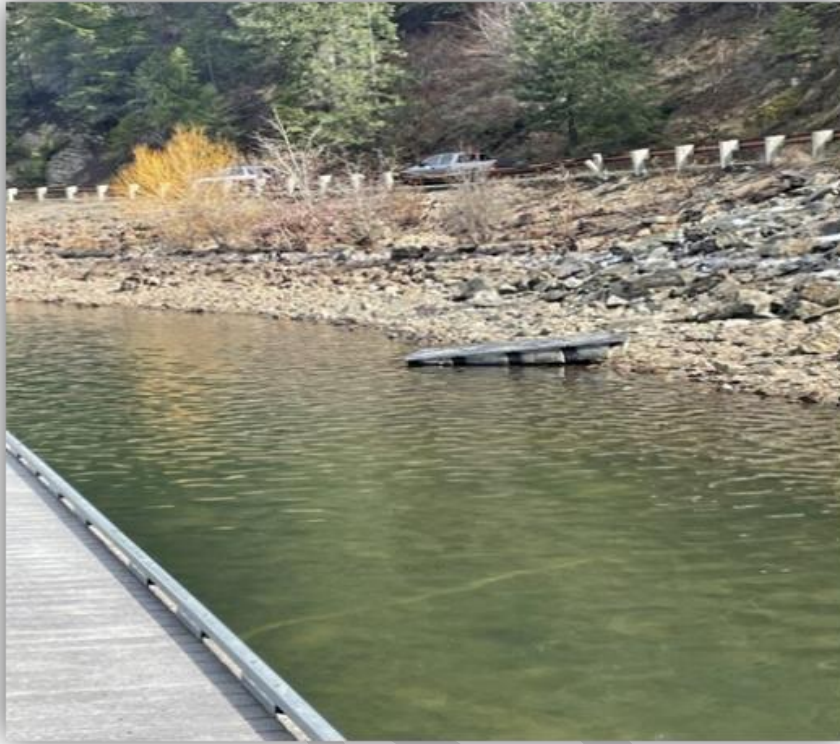
Figure 9: Dislodge dock float tub at Mineral Ridge Boat Launch
