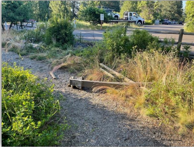
Figure 8: Damage to Fence and Native Plant Garden from runaway vehicle
