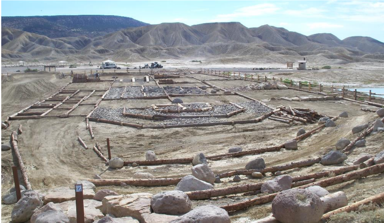
Peach Valley OHV Skills Course – Construction Phase
