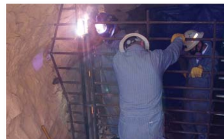
Closing one of many mine openings in the Cottonwood Wash area.
