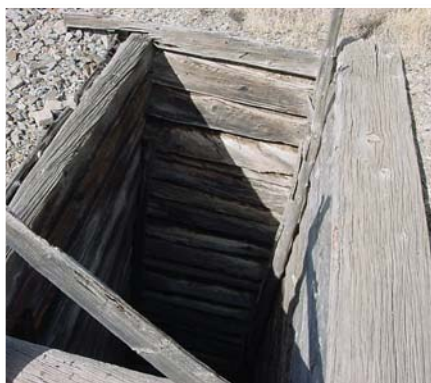
One of several open vertical shafts addressed at the Reef Gulch site in Colorado.
