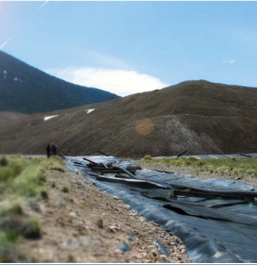
The Golden Butte Mine site in Nevada.
