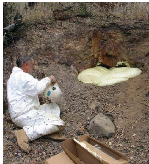
Foam closure at the Humbolt Mine.
