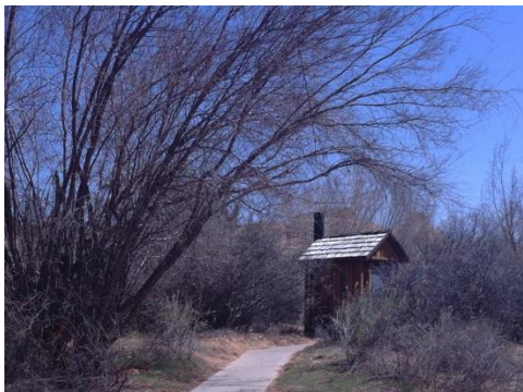
Deer Creek pit toilet
