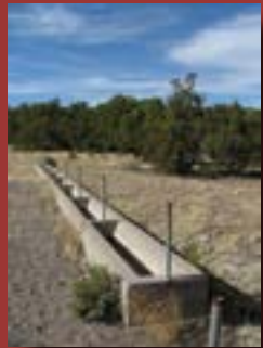
Example of a trough installed by the CCC—this one is at BLM's Datil Well Campground.
