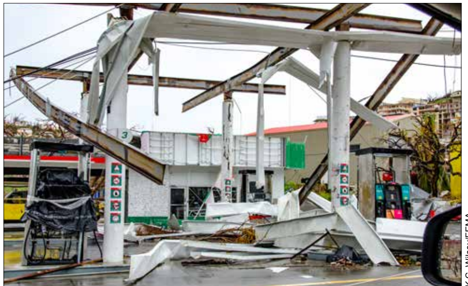
Steel girders and torn sheet metal are all that remain of the structure that covers the fuel tanks at a local service station on St. Thomas. The force of the winds from Hurricane Irma ripped apart this gas station in Charlotte Amalie.
