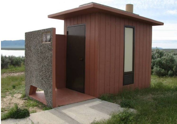
Figure 8: Repainted vault toilet at Wilson Campground
