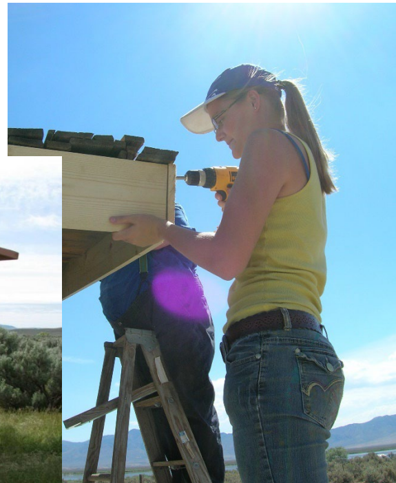
Figure 6: Work on kiosk funded by FLREA fees
