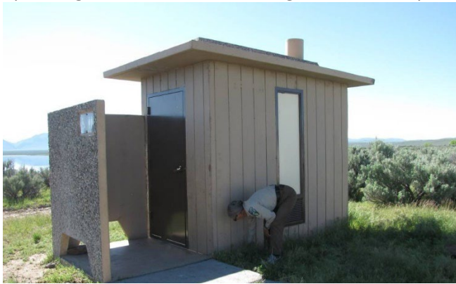
Figure 7: Before painting of single vault toilet at Wilson Campground
