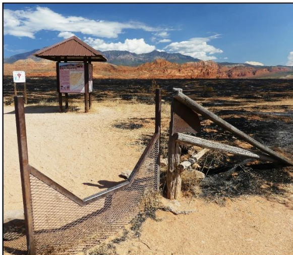
Figure 1: Cottonwood Trailhead fire damage.
