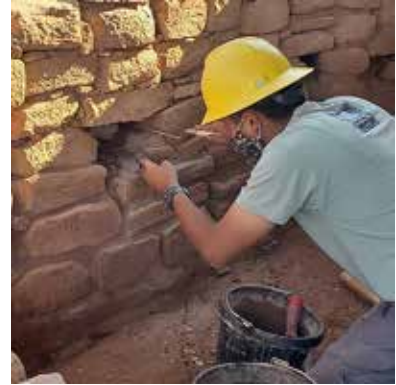
The Southwest Conservation Corps' Ancestral Lands youth crew assisted a professional stabilization crew at a prehistoric masonry pueblo at Lowry Pueblo National Historic Landmark.
