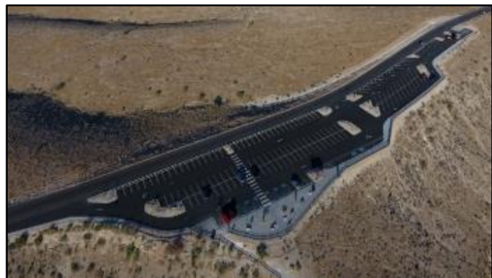
Figure 4 Calico I Expansion
