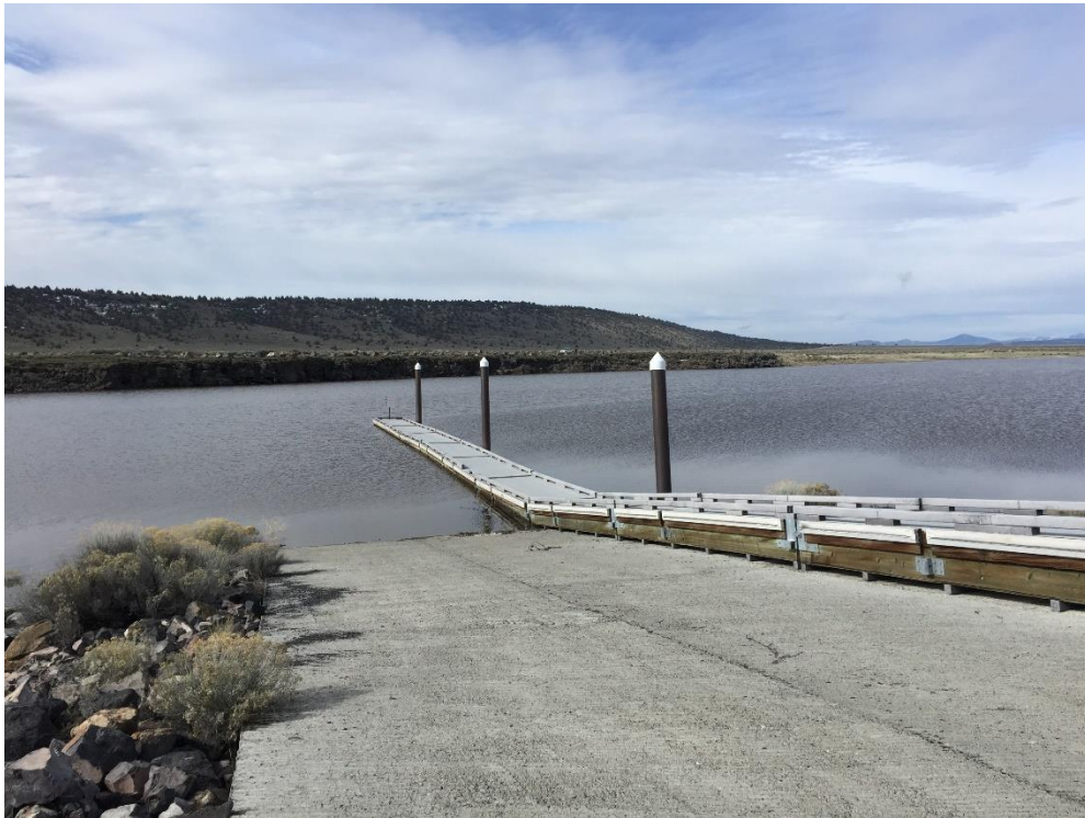
Boat ramp and floating dock
