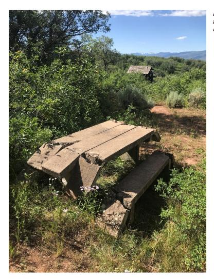
Figure 2. Concrete picnic table: one of three identical tables to be historically reconstructed.
