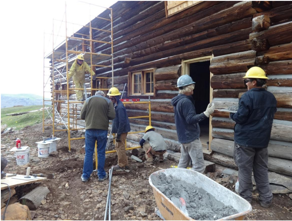
Golconda Boarding House during restoration by Colorado Youth Corps members.
