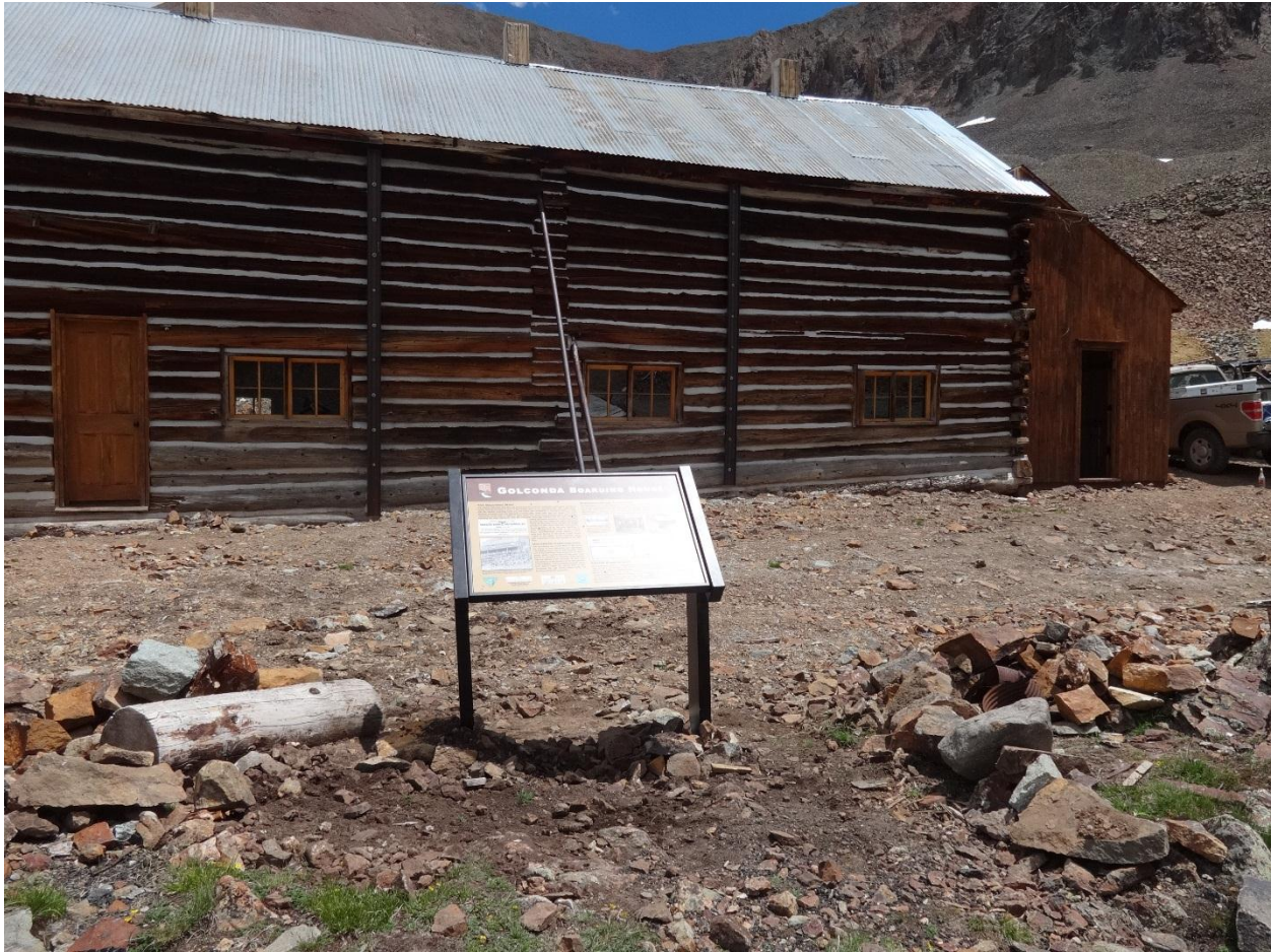
Golconda Boarding House after restoration with newly installed interpretive panel.
