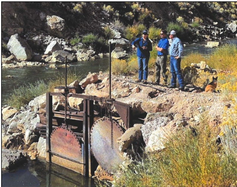
Figure 3. Headgates of the Maybell Ditch.
