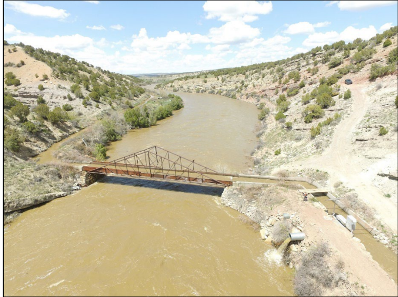
Figure 2. Aqueduct transporting Maybell Ditch water across the Yampa River.
