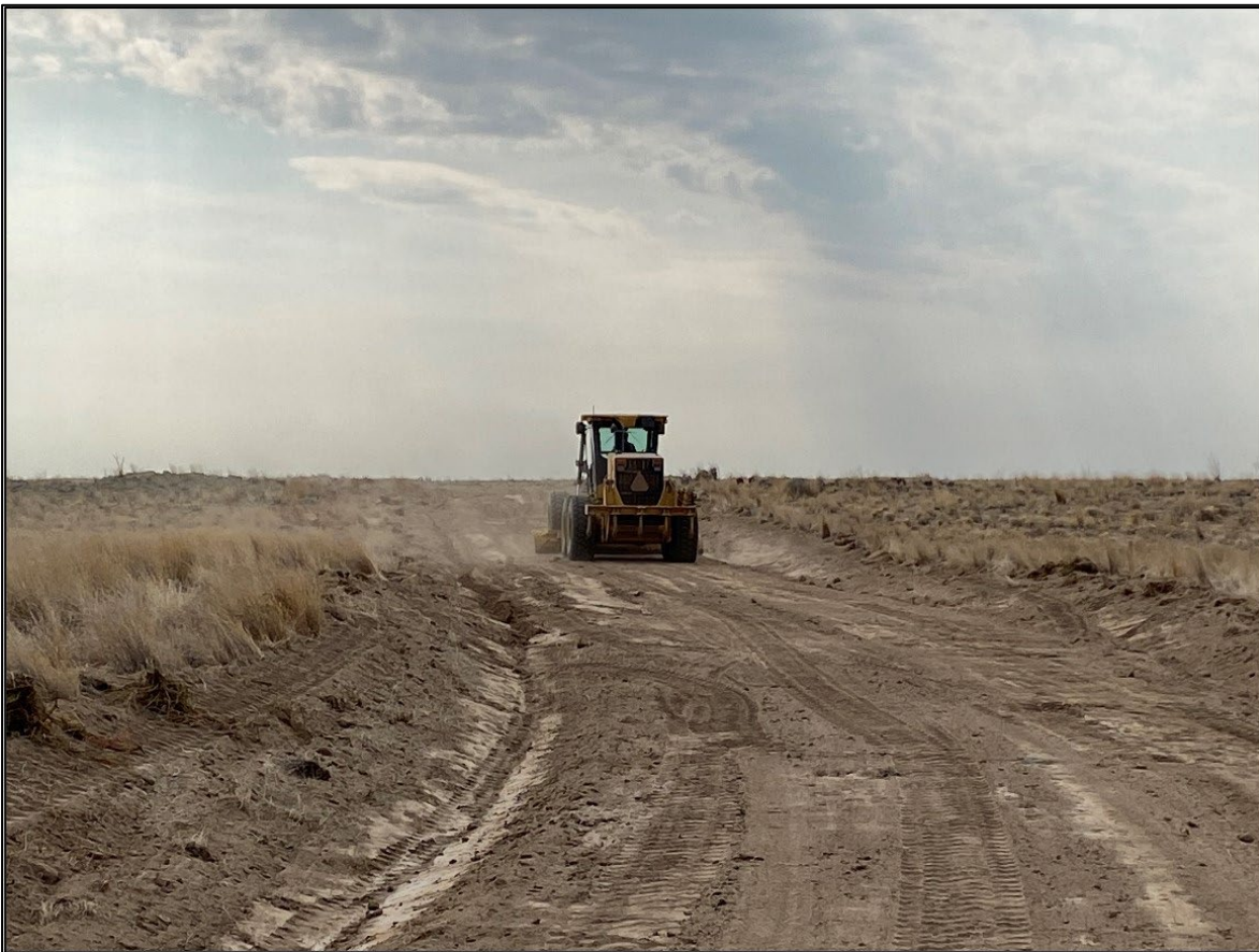
Road work on the Arco-Minidoka Road
