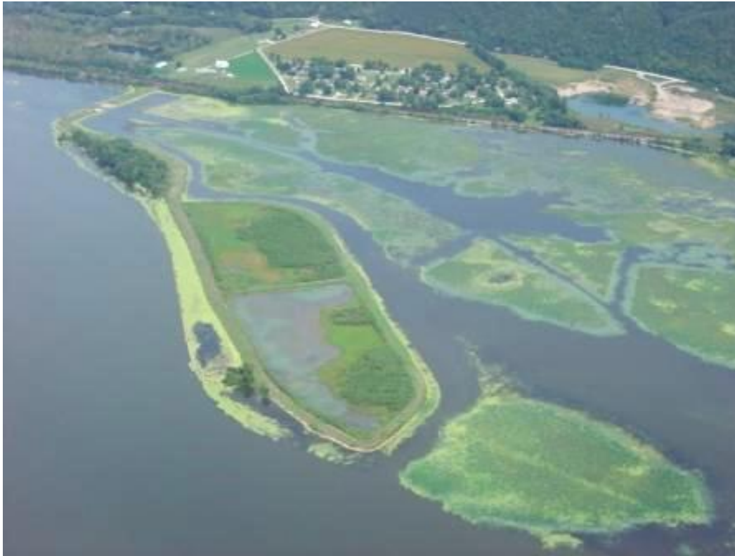
Photo. RIVERS ALSO NEED NATIVE SEED. Upper Mississippi River Restoration Environmental Management Program of US Army Corps of Engineer. Credit: Rock Island District (army.mil)
